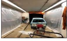
4. Ready to get some prep going ?...Sand all surfaces with 80 grit sandpaper using either, hand, orbital sander or wire brush grinding to etch all coating surfaces. THIS IS YOUR "KEY" TO
